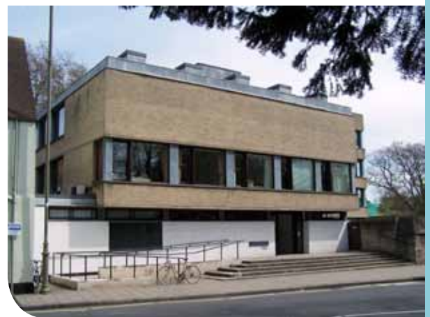
St. Giles' building
